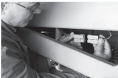
**Phase 5:** Connect one of the 6 mm<sup>2</sup> conductors to a fuse 40A (absorption 23A), then connect the second conductor to the ground. If greater length is required, use a 10 mm<sup>2</sup> conductor.
