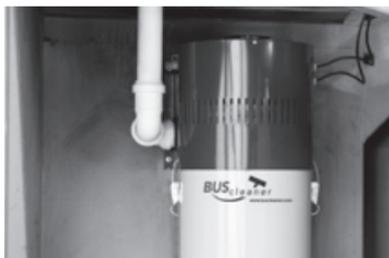
**Phase 3:** Connect one end of the tube/hose to the vacuum cleaner and the other to the socket.
