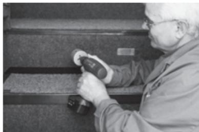
**Phase 2:** Fix the suction socket to the 3rd step using a hollow mill (60 mm).
